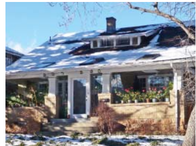
This glass enclosure is a non-invasive strategy for a weatherization improvement. It captures winter heat on a front porch, while retaining the building's historic character and materials.
