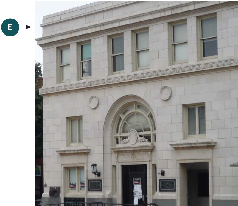
Protect and maintain significant stylistic features, such as these window features, cornice details and ornaments.
