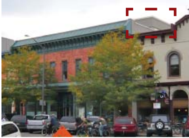
This photo also shows an appropriate addition where the roofline is altered but is not very visible from the public right of way.
