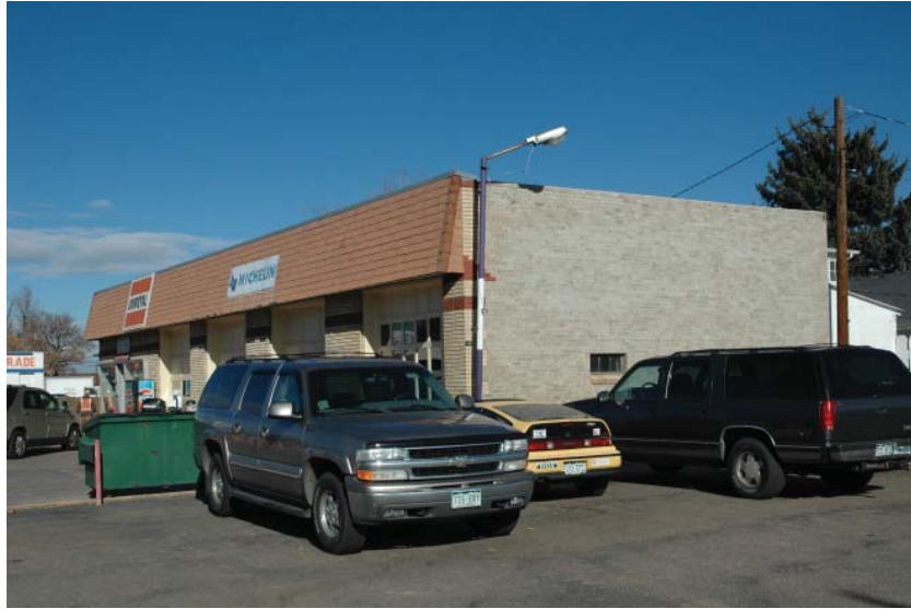
CD 2, Image 1, View to NE of façade (west) and south side
